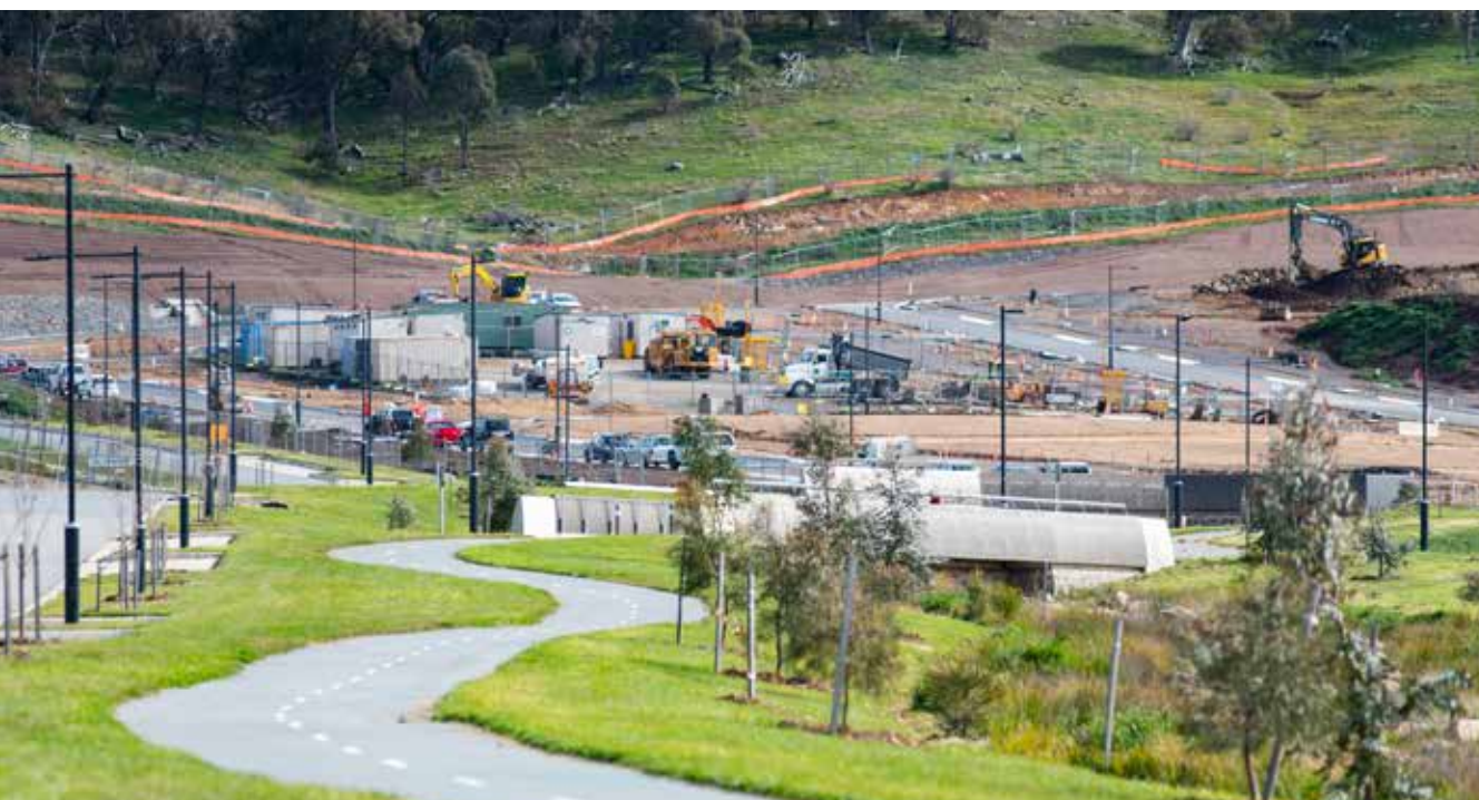
◀ Taylor under construction
